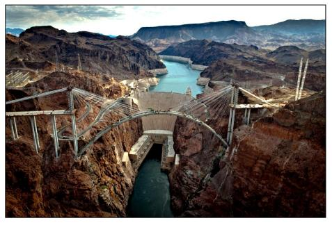
When complete, it will provide a new link between the states of Nevada and Arizona. In an incredible feat of engineering, the road will be supported on the two massive concrete arches which jut out of the rock face.
