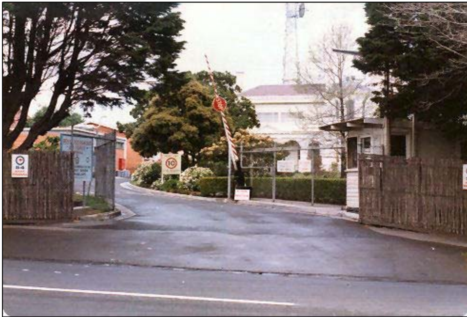
The main gate, with the Head Quarters building in the back ground.
