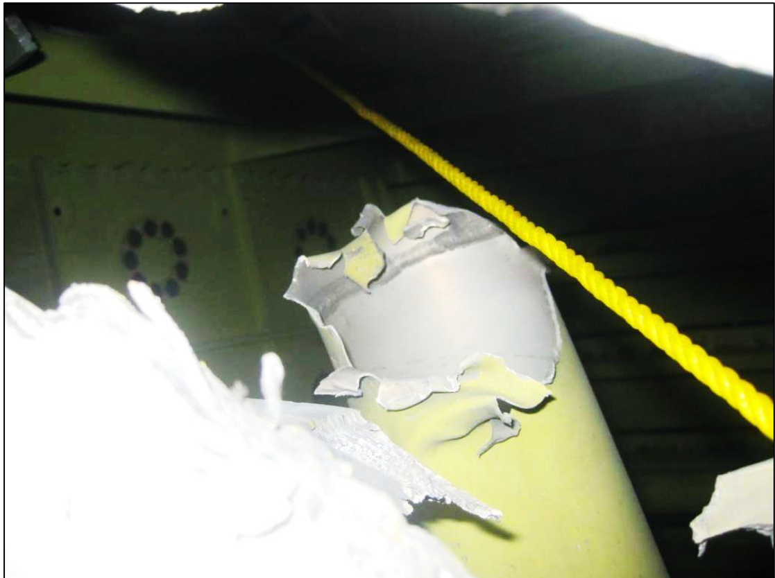
Figure 8: Severed fuel pipe at frontspar/Rib 9
