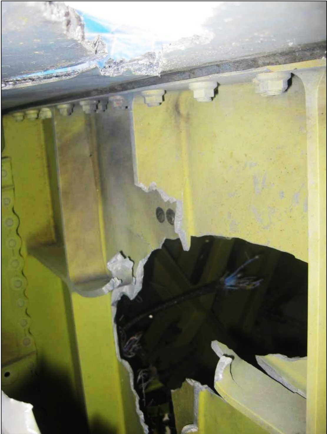
Figure 9: Section of front spar damaged view in aft direction)
