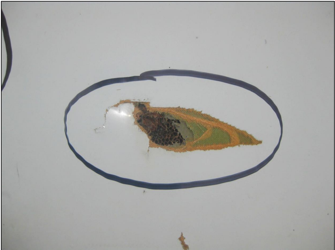
Figure 13: Skin perforation showing honeycomb
